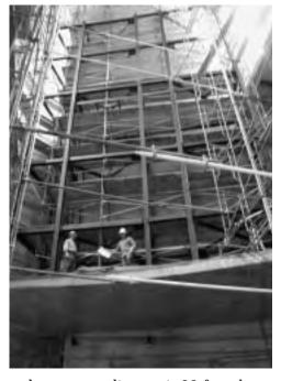
ment. The platform they are standing on is 20 feet above the raised choir level, with the steel framework topping out 53 feet overhead. The instrument will be enclosed in an American cherry case 58 feet tall, 33 feet wide, and 11
