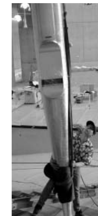
Uwe Dohrmann, foreman from Giesecke, steadies 32' D in its sling as it is hoisted into place.
