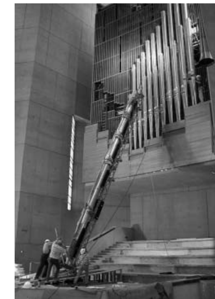
Using a support cradle, 32' C# is muscled into vertical position
